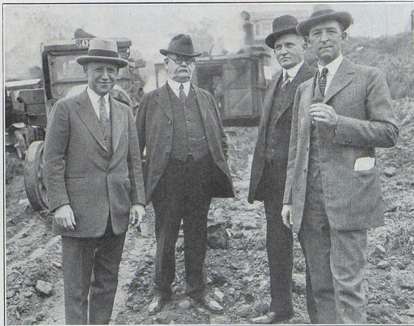
Four leaders and active participants in great underground bore. Left to right—E. C. Johnson, Chief Engineer; Judge John Twohy, Contractor-in-chief; D. W. Pontius, Vice-President & General Manager; W. R. Fontaine, Consulting Engineer associated with Twohy Brothers.
