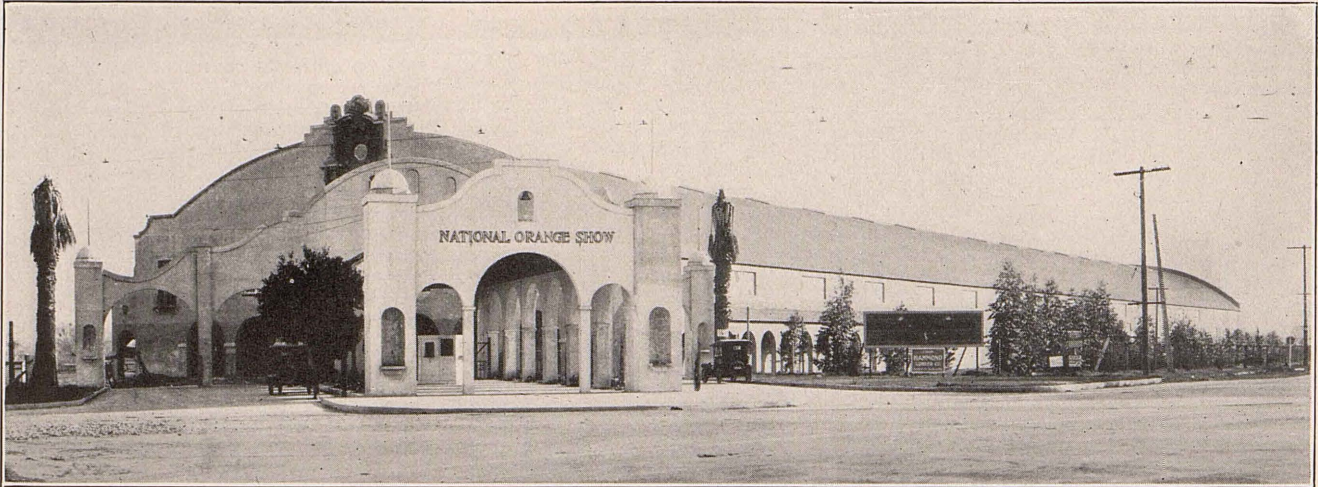
Visitors to the National Orange Show this year will be agreeably surprised and pleased with the large permanent home of the Orange Show. The building is more than 700 feet in length and about 200 feet wide.
