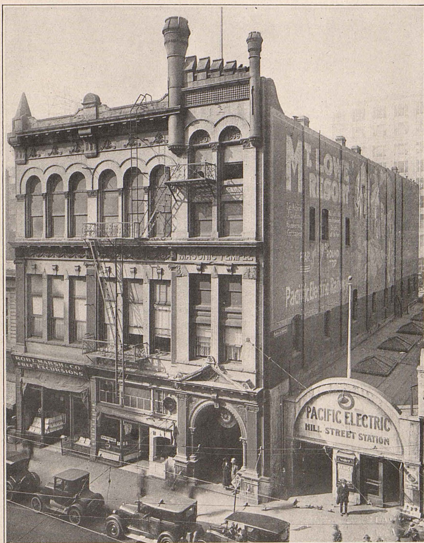
Razing of the familiar old landmark shown above was begun January 6th to make room for the temporary station to be used pending the construction of Terminal Subway Building.
