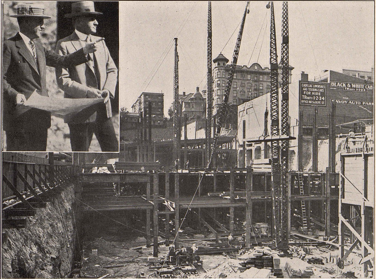
Structural steel workers are maintaining the same dizzy pace that has characterized the progress of other crews on terminal and tunnel project. Vice-President Pontius and Chief Engineer Johnson are seen on a tour of inspection.
