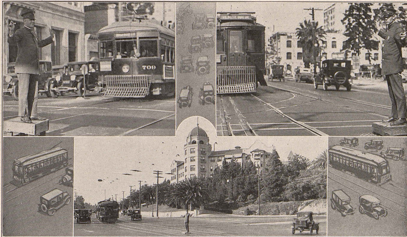
No small part of the success of handling immense traffic volumes on the streets of Los Angeles may be attributed to the efficiency of the city's able traffic officers. The pictures presented show Officers C. F. Jetton (left), J. Annas (right), and G. R. Mitchell, below, "doing their stuff."
