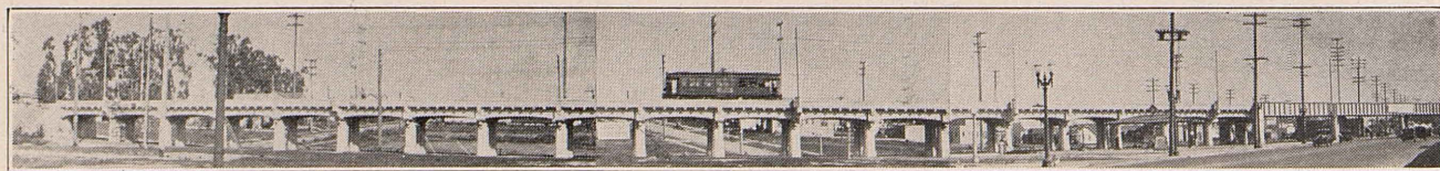
A good conception of the length and pretentiousness of the Pico Street grade separation is obtained from the above photograph. The structure measures 1007 feet in length. The absence of noise and rumbling is a feature that has attracted widespread attention.
