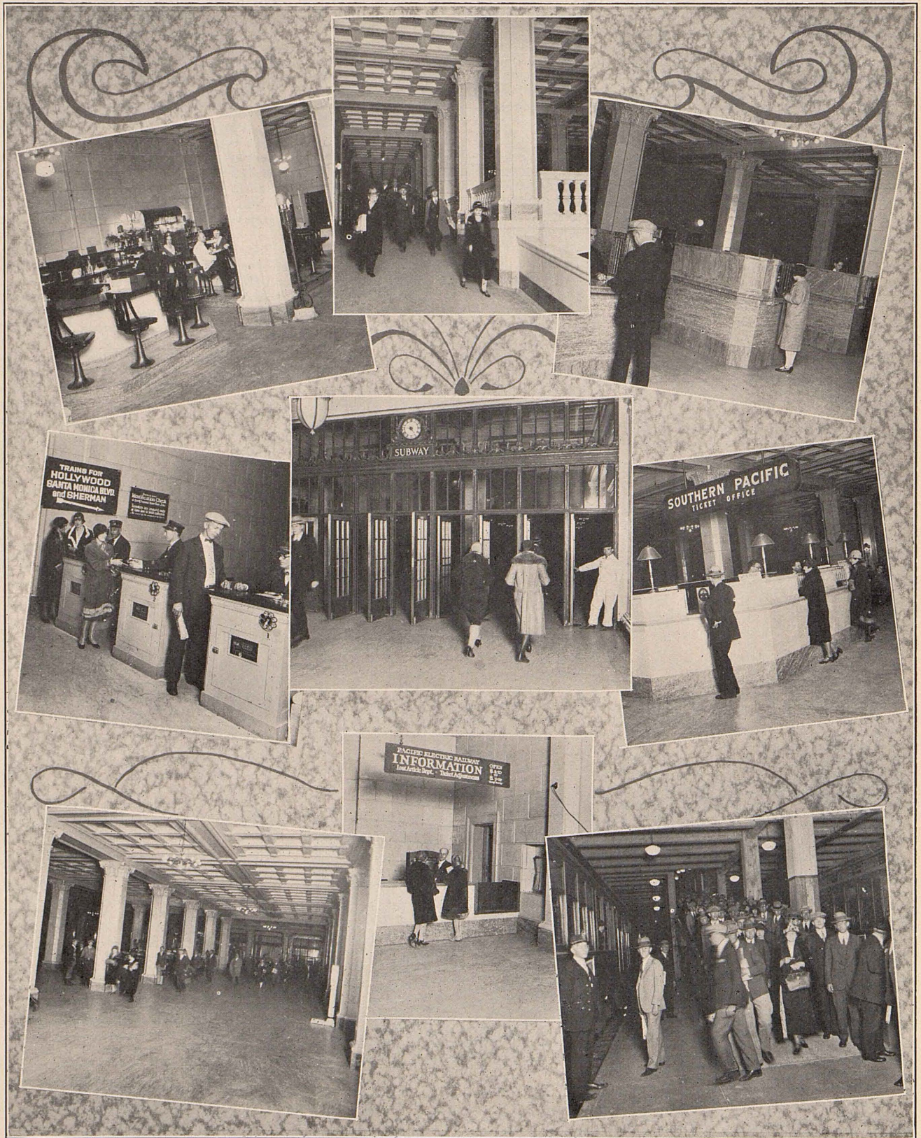
Familiar Views in New Subway Terminal Station Where Facility is Provided for Rapid and Comfortable Handling of Patrons Destined to Points on Western Division. Note High Class of Architecture Employed.
