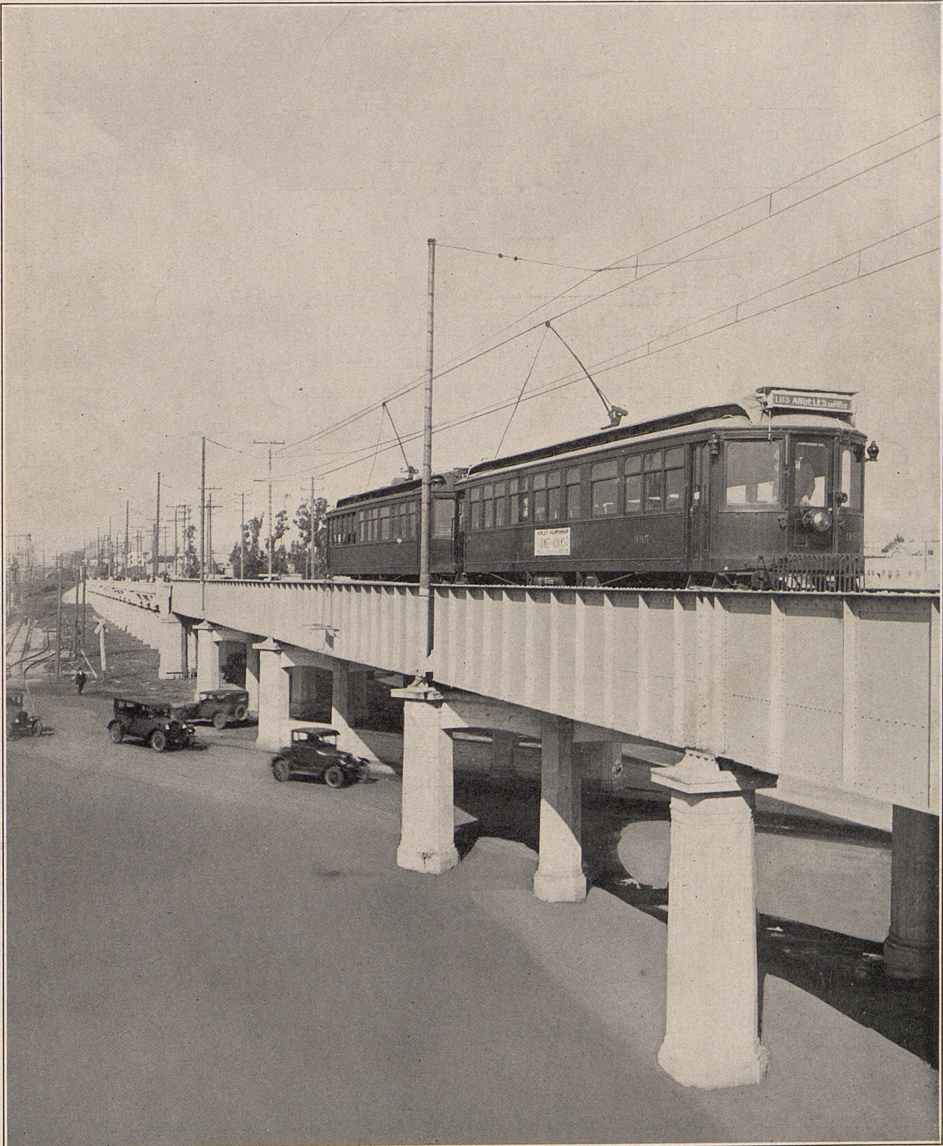
Pico Grade Separation, Now Nearing Completion
