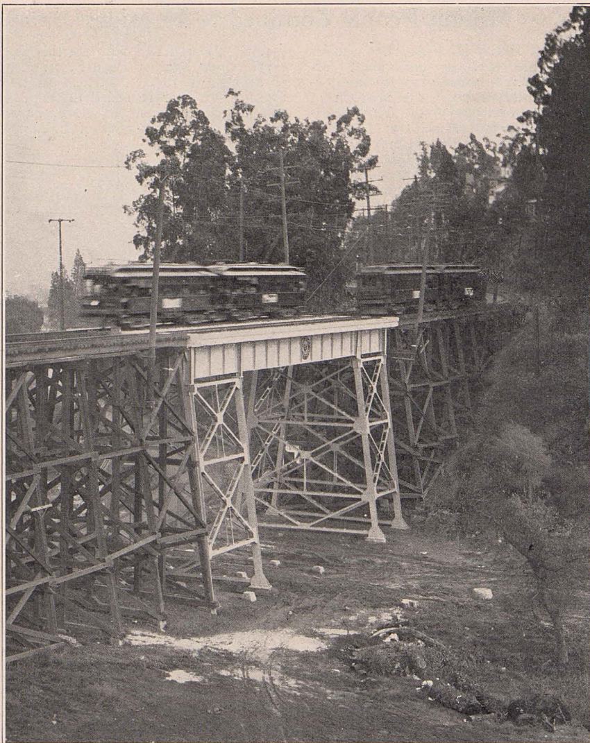
Steel span structure recently completed by our Bridge & Building forces over Fletcher Drive, soon to become a great artery of travel to Glendale and Burbank districts.
