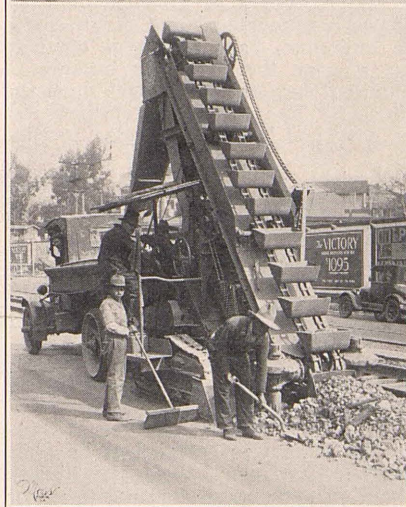
Speeding up and lowering of costs will result from recently acquired electrically operated shovel and loader now being employed by Engineering Department forces.
