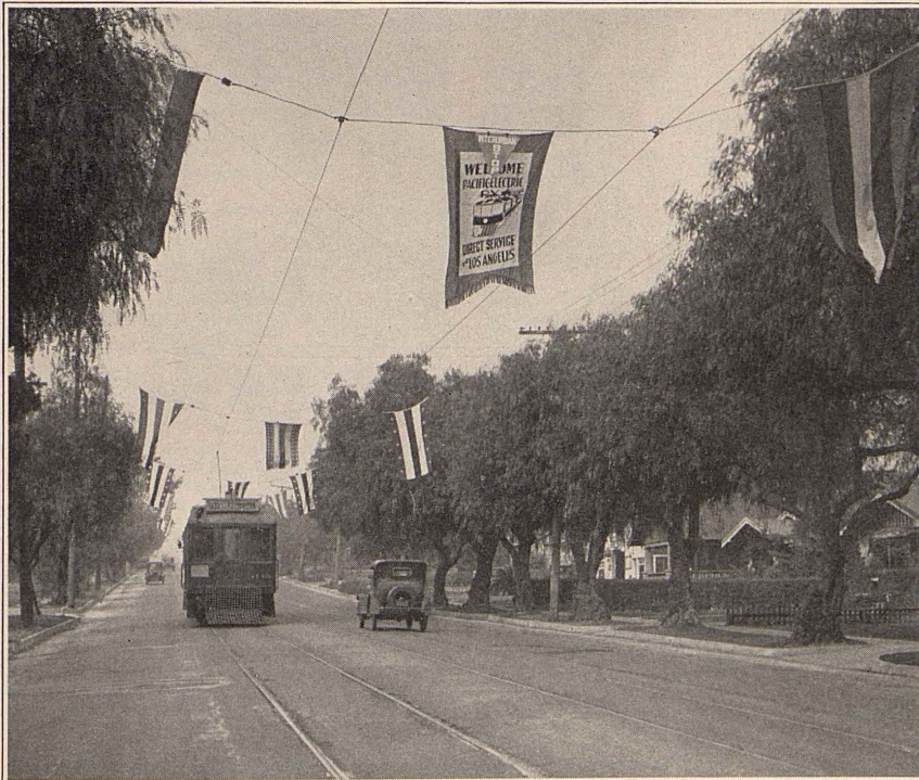
Altadena and adjacent districts know the value of direct interurban passenger service. "Welcome Pacific Electric" read many suspended banners amid a civic celebration held commemorating the re-routing of Oak Knoll line trains to the new terminal on Lake Street.
