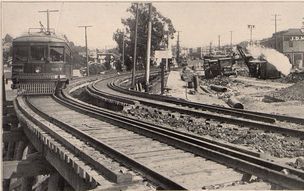
The projection of Myra Street under Sunset Boulevard necessitated removal of tracks to a bridge shoo-fly pending construction of concrete structure across Sunset. Such jobs are "just another day" to Engineering Department forces who completed the detour in short order.
