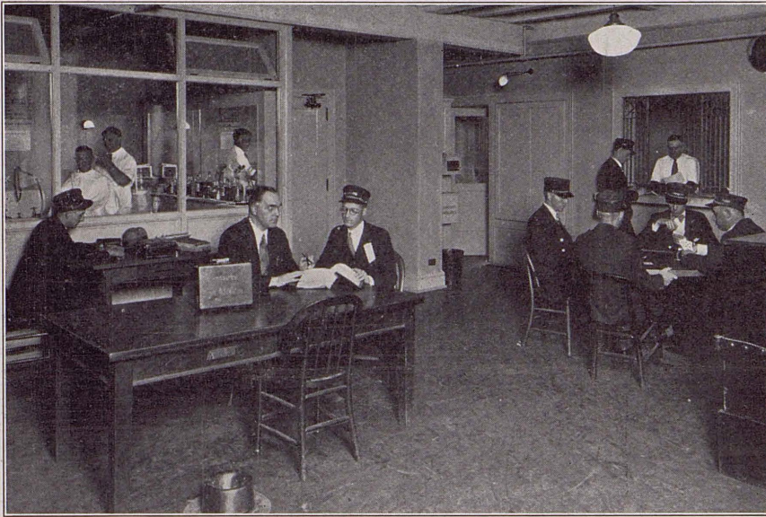
Convenient both to the yards and viaduct the new Trainmen's quarters in the Club building is well filling the needs of the five hundred Trainmen who work out of the Main Street Terminal.
