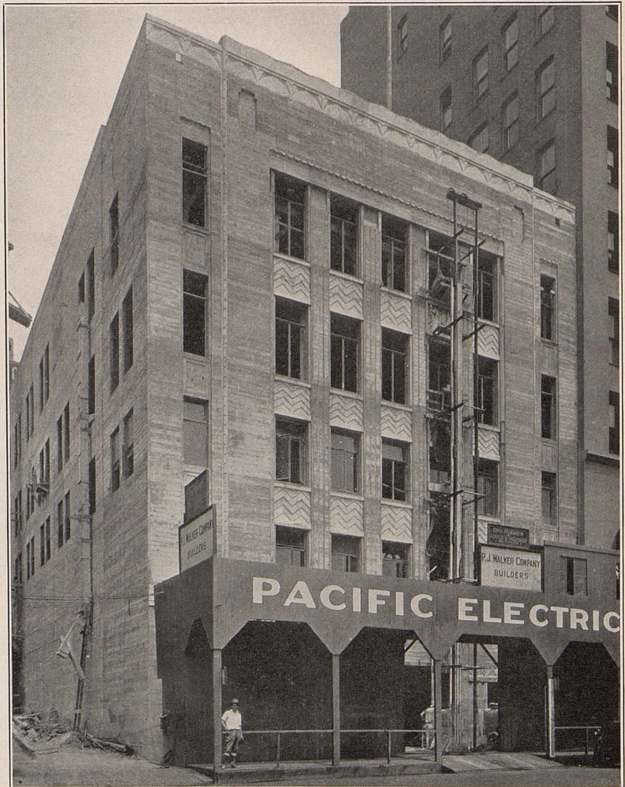
With inside finishing on our new Club Building progressing at a rapid pace, as is plainly evident from the fact that windows have been placed in the lower floors, assurance is given that "it won't be long now." Note the artistic architecture.
