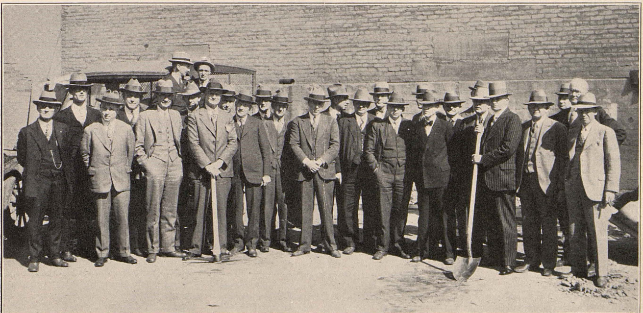
Just a few moments after this picture was taken a steam shovel nosed into the earth and construction of new club building was on in earnest. The group are officials who participated in ground breaking ceremonies celebrated on Friday, February 15th.
