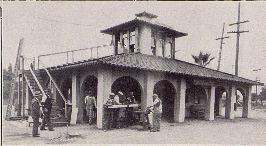
Views of Main Street (left) and Oneonta interlocking plants, both of which are among the seven which have been modernized to the highest degree of efficiency.
