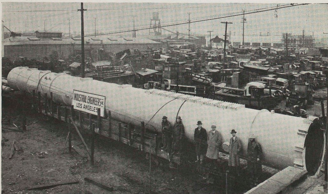
A 92-foot fractionating tower, requiring three flat cars and good railroading to transport, arrived in good order at Maricopa, originating at Wingfoot district. It was 7 feet in diameter and weighed 49 tons. Starting third from left: Wally Hickman, S. P. freight department; Dave Porter, P. E. freight solicitor and G. P. Barkhurst, Agent at Wingfoot. Rubber clad gents are members of train crew.
