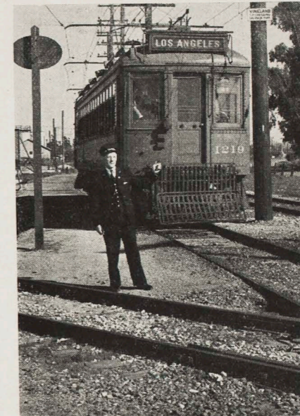
WRONG WAY Conductor has not crossed tracks or observed steps to see if any passengers are boarding or alighting.
