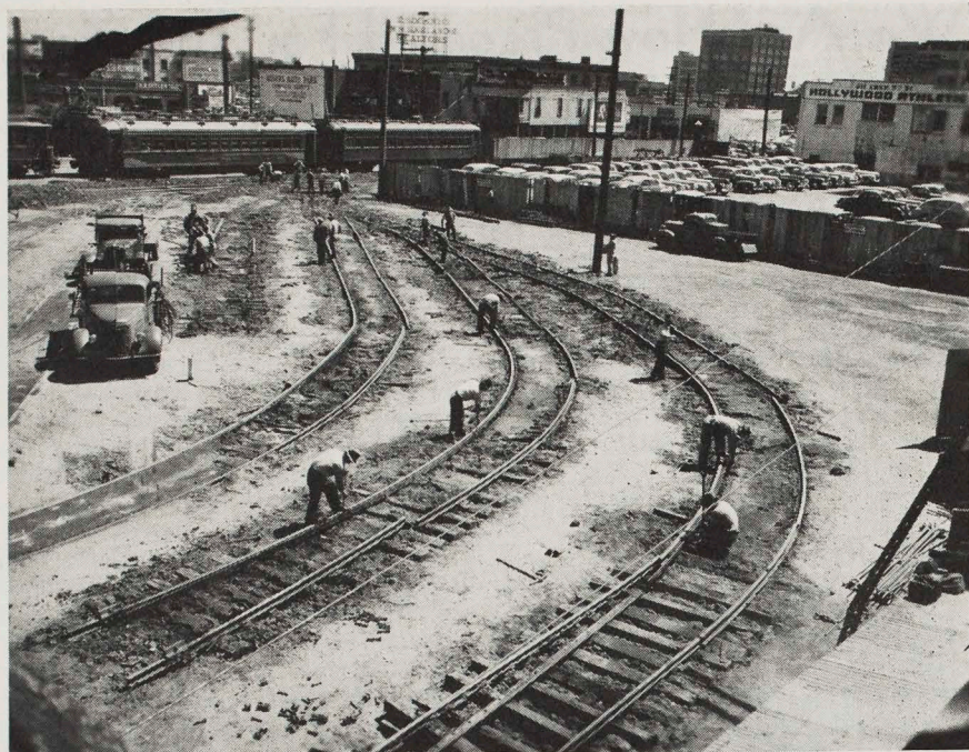
Tearing out tracks in the Los Angeles Street Yards to make room for New Coach Garage that will extend over most of the area shown. Two tracks will remain between Sixth and Seventh Streets to serve U. S. Mail and Express interests. Entrance to the garage will be from Maple Avenue, past the present servicing and running repair shop.
