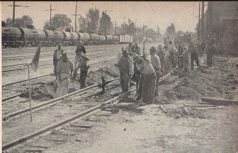
SECTION GANG working at San Bernardino yard.
