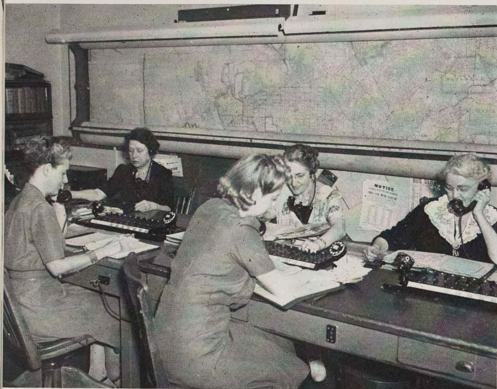
CLIMBS SKYWARD —The Information Switchboard has moved from the fourth to the seventh floor of the P. E. Building. Left to right: Catherine Rebold (Mrs. Ed Haldeman), Edna Tilley, Doris Burden, Deane Aspelmeier, and Chief Sybil Mather. Note the huge wall map of the city.
