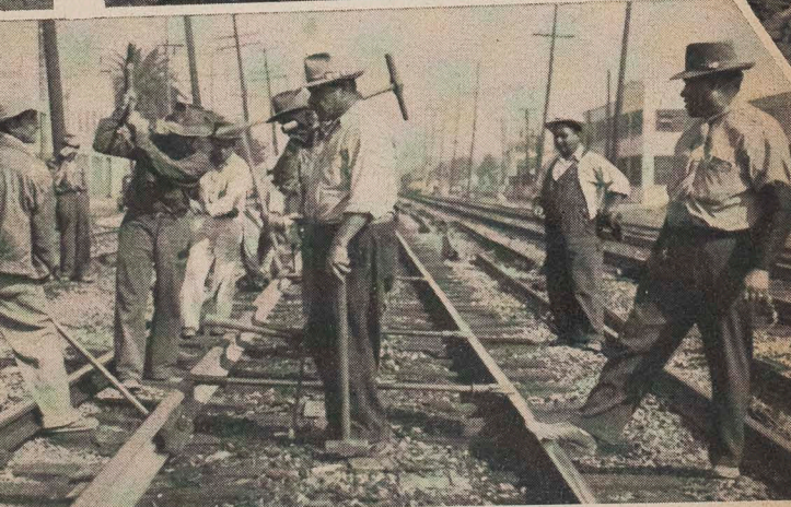
HOW THEY DO IT —L. H. row, top to bottom: Navajos work on West Basin. Planer blade smooths paving softened by heat from planer. Foreman W. Chappell (white gloves) & M. Cook (vest) combine gangs for job. Ex. 8 raises track with spotboard. R. H. row: Ex. 2 lifts rail into place ("Arriba!" — "Up!"). Gravel train backs up & spreads dumped ballast. Ex. 2 Foreman B. Leyva (extreme right) supervises laying 90-lb. rail, using track gauges. Center bottoms William F. Shea, special assistant to Mr. McClure.
