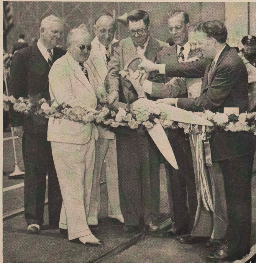
ALISO STREET VIADUCT OFFICIALLY OPENED to highway traffic on August 14 with the cutting of this rope of asters by a pair of five-foot shears. Having a hand in the cutting were, left to right, City Engineer Lloyd Aldrich, Mayor Fletcher Bowron, Councilman J. W. Baumgartner, President O. A. Smith of Pacific Electric, Chairman Herbert C. Legg of the Committee for Congested Production Areas, Harrison R. Baker of the State Highway Commission, and Supervisor John Anson Ford. Pacific Electric trains have been crossing the viaduct since July 18, 1943.
