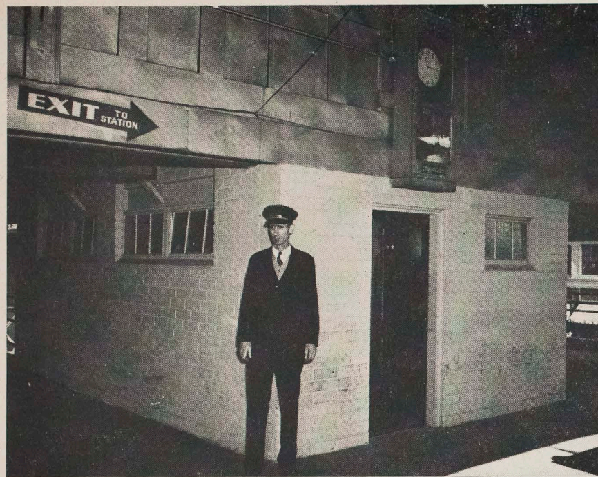
NEW CASH RECEIVING OFFICE on the Sixth & Main Viaduct was completed last month to replace the old, inadequate one just across from it. The new one, besides providing more commodious quarters for the Cash Receivers, has the receiving windows inside where Conductors are not disturbed by noise, wind, and the jostling of passengers rushing to their trains. The trainman in the picture is P. J. Bever—who, incidentally, in his nine years with P. E. has qualified as Dispatcher, Motorman, Conductor, Operator, Terminal Foreman, Stationmaster, Freight Motorman, and Fireman.
