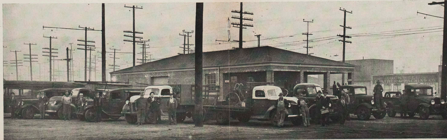
NEW SIGNAL & BONDING STORE at Washington Street Yard, with Signal and Bonding trucks backed up against the loading platform. The store was opened on September 18, when the scene of Signal Department operations was shifted to Washington Street. Considering that this pan-
