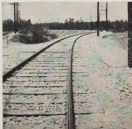
SHOOFLYS had to be built at San Bernardino on the government storm drain project now in progress. The two pictures at left show (top) shoofly at Bethune before main line was cut over to it, and (below) shoofly installed. The two pictures at right show (top) main line at Bench being cut over to a shoofly, and (below) shoofly installed. Extra Gang 9, with Tom Sharp as Foreman, did the work on both shooflys.
