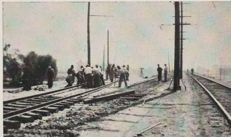
SHOOFLYS had to be built at San Bernardino on the government storm drain project now in progress. The two pictures at left show (top) shoofly at Bethune before main line was cut over to it, and (below) shoofly installed. The two pictures at right show (top) main line at Bench being cut over to a shoofly, and (below) shoofly installed. Extra Gang 9, with Tom Sharp as Foreman, did the work on both shooflys.
