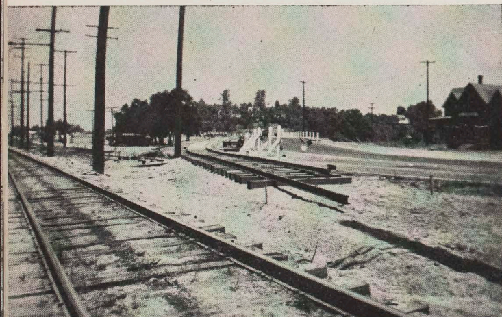
SHOOFLYS had to be built at San Bernardino on the government storm drain project now in progress. The two pictures at left show (top) shoofly at Bethune before main line was cut over to it, and (below) shoofly installed. The two pictures at right show (top) main line at Bench being cut over to a shoofly, and (below) shoofly installed. Extra Gang 9, with Tom Sharp as Foreman, did the work on both shooflys.
