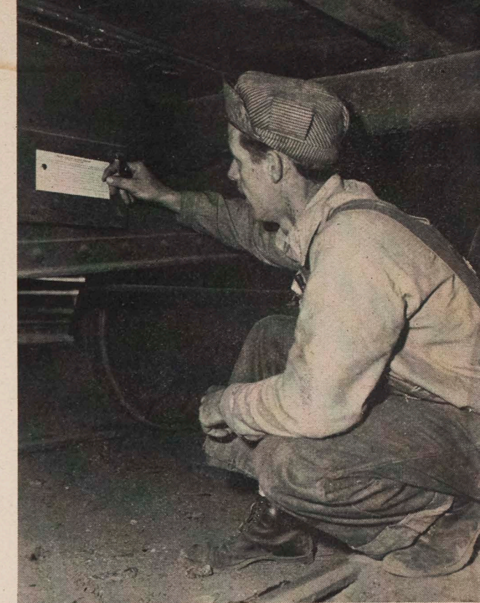
CAR INSPECTORS are located at interchange points and other strategic points on the PE freight system to see that cars are in proper condition. Immediately upon the arrival of a train, the Car Inspector inspects every car and makes such minor repairs as are necessary. Heavier repairs are made at the Butte Street rip track. Car Inspectors also look for defect cards on cars that come in from other lines, as Roy Hegglin of Butte Street is doing here. If a foreign-line car is so badly damaged as to require major repair work, it is usually given enough care to enable it to be sent back to the owning line, which is billed for work done. Car Inspectors may also be called in to inspect a load in cases of doubt that a car is properly loaded.
