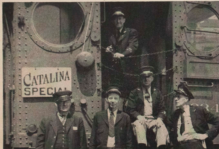
CATALINA SPECIAL CREWS from Los Angeles and from Long Beach: The Los Angeles crew consists of G. G. Caldwell, Head Conductor, extreme right; Jack ("Half-Pint") Eastwood, Motorman, next to Mr. Caldwell; and A. M. Engle, TrILERMAN, extreme left. The Long Beach crew consists of H. A. Wilkerson, Head Conductor, leaning on chain; S. E. Matheny, Motorman, second from left. "Cowboy" Cox took this picture shortly after the resumption of Catalina service. Catalina travel has so increased that more cars and more Trainmen have been added, and several of the men pictured have changed jobs.
