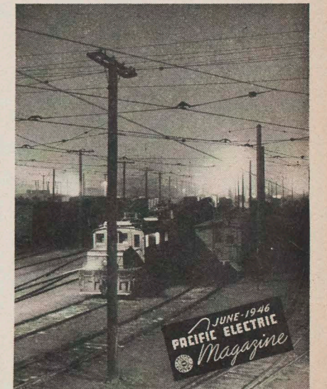
COVER PICTURE Butte Street Yard at Night
