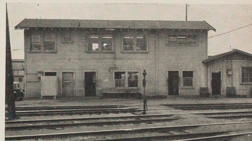
BUTTE STREET YARD OFFICE
