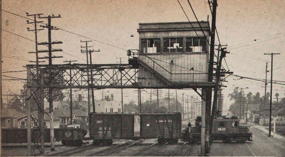
Train from Santa Monica Air Line heading east into Butte Street Yard and crossing the Four Tracks at Amoco Tower.
