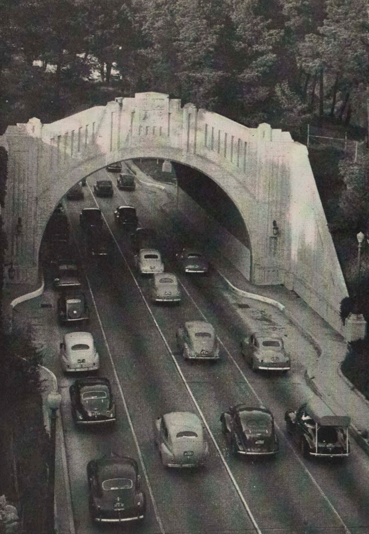
HEAVY TRAFFIC flows easily through the Figueroa Tunnels .
