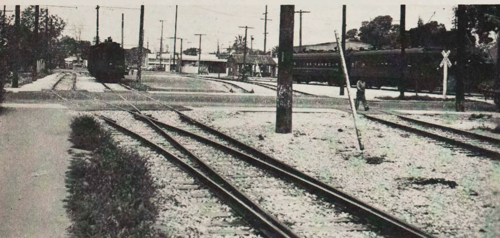
NEW SANTA ANA YARD — Above, looking north on new yard recently placed into service at Santa Ana Station. The skeleton building, soon to be completed, is the new quarters for Trainmen. Below, the old team track formerly down the center of the bus lot has been removed to make room for busses, and to facilitate their loading. Trains now swing further around the bus lot to come into the new yard.
