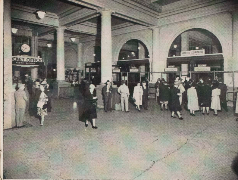
BUS GATES: left, before, and right, after alterations. Compare also old beamed ceiling with new flat ceiling;
