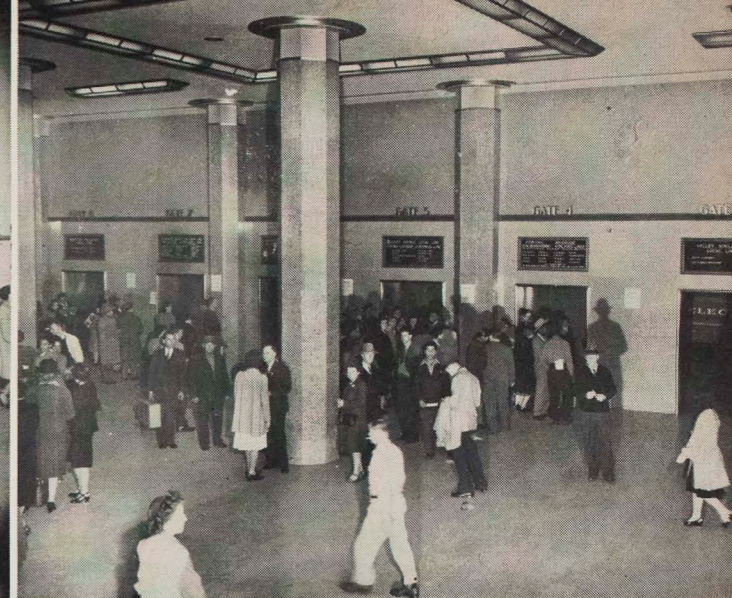
old chandeliers with new fluorescent lights; old round pillars with massive bases with new octagonal pillars.
