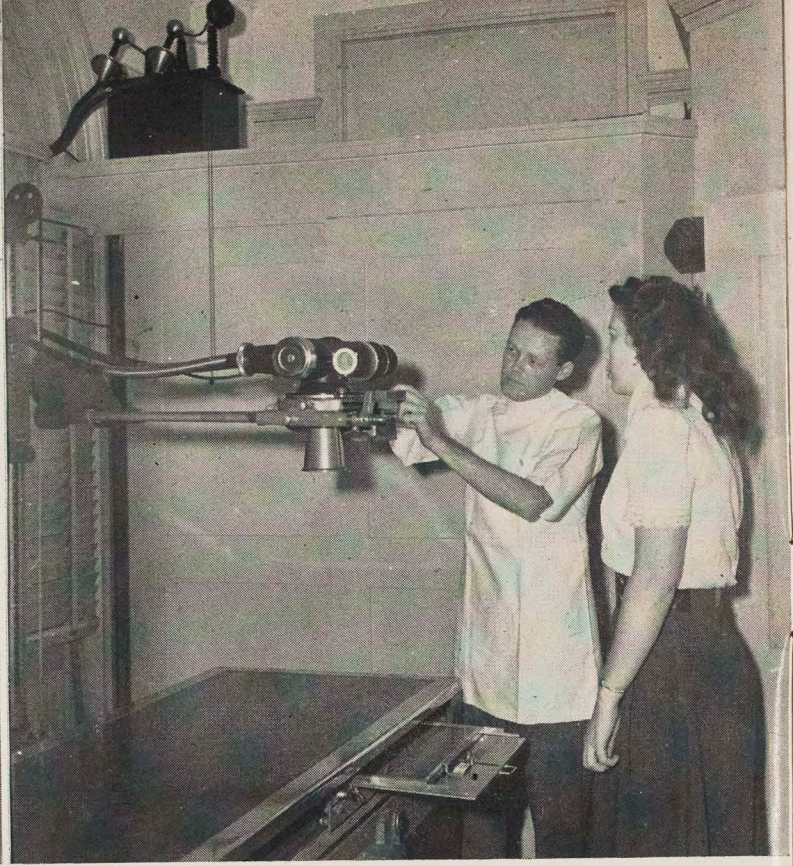
NEW TUBE , shock proof and air blower cooled, is explained by Technician Archie Lineer. It replaces an obsolete tube. New transformer at upper left permits simultaneous use of this room and therapy room.
