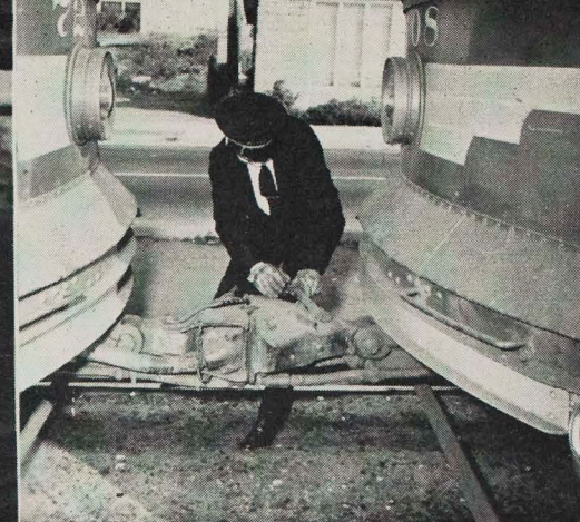
15. At the east switch he uncouples the two cars. Head car moves on, leaving Car 708 just east of the switch, for easy handling.
