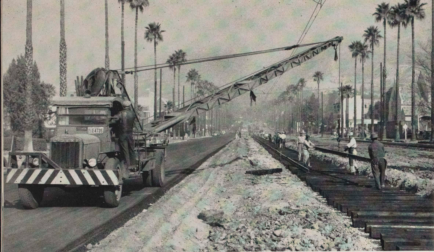
GENERAL VIEW of North Brand project as of about Dec. 1
