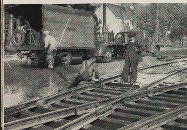
LEFT, Bonders and Welders at work on North Brand project. RIGHT, and Alexander Paul (right), Foreman of Section No. 7. Section men laid the new track in record time, as all rail traffic was stopped.
