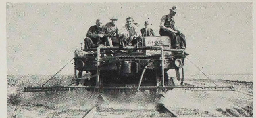
NEW WEED-KILLING EQUIPMENT, the Hykil T-80 Sprayer, developed by the W. T. Cox Co. of Santa Ana, was given a trial run Nov. 22-23 on the Stanton-Los Alamitos and the Stanton-Huntington Beach lines. Ball joints on the spray pipe enable the equipment to pass line poles. Heart of the machine, which may be installed with relative ease on a flat car, is a gasoline-driven pump which emulsifies and pressurizes oil and water. Gauges indicate the exact amount of oil and water used on a run. Use of several valves makes it possible to shut off sections of the spray pipe at will. Witnessing the demonstration for PE were H. J. Culp, Paving Foreman, and L. J. Bush, Roadmaster. Train Crew included I. C. Colt, Engineer; G. K. Herbold, Conductor; C. E. Saylor and J. R. Norte, Brakemen; and F. P. Fitzpatrick, Trolleyman. Left to right in picture are W. T. Cox, Mr. Herbold, Edwin Cox (who operated the sprayer), Mr. Culp (hat only shows), Mr. Bush, and Thomas M. Cox.
