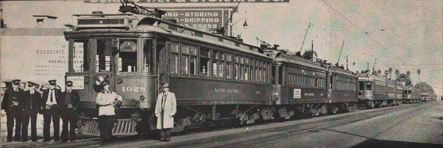
LINED UP FOR BLOCKS on Fair Oaks Ave., south of Colorado St. in Pasadena, were trains like these awaiting to be dispatched at 10-minute intervals back to Los Angeles after having brought their loads
