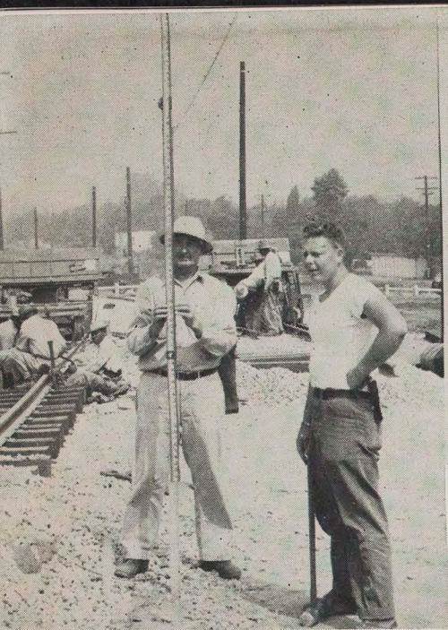
SETTING LINE AND GRADE STAKES for rail on bridge are Rodman Robert G. Aten, left, and Junior Engineer (i.g.) A. R. Strople.
