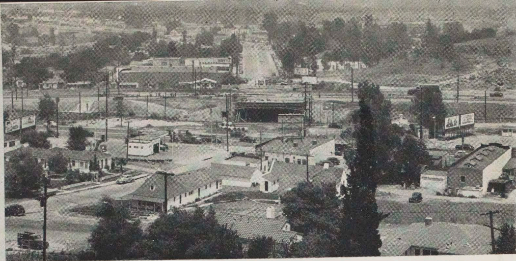
BIRD'S-EYE VIEW of Lankershim grade separation project, Universal City, at Lankershim and Cahuenga Blvds., looking north. New PE tracks over bridge will eliminate dangers of heavy highway traffic on Lankershim. Old rails parallel Cahuenga Blvd., at street level.
