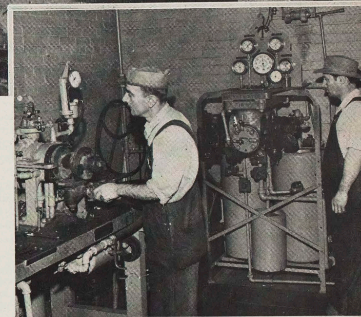
ABOVE: Overall view of Air Room, where air brakes are repaired.
