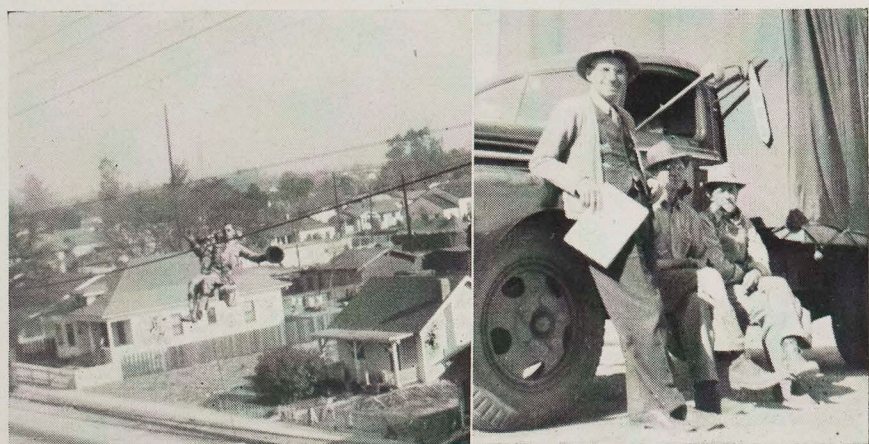
SIGNALMEN —Between earth and sky in picture at left is Darold E. Burleigh, riding a cable car while working at Graham Yard. In picture at right are, left to right, Foreman Felix Brac, Signalman Floyd Benoit, Signal-Wireman Roy Steed, snapped working at Watts.
