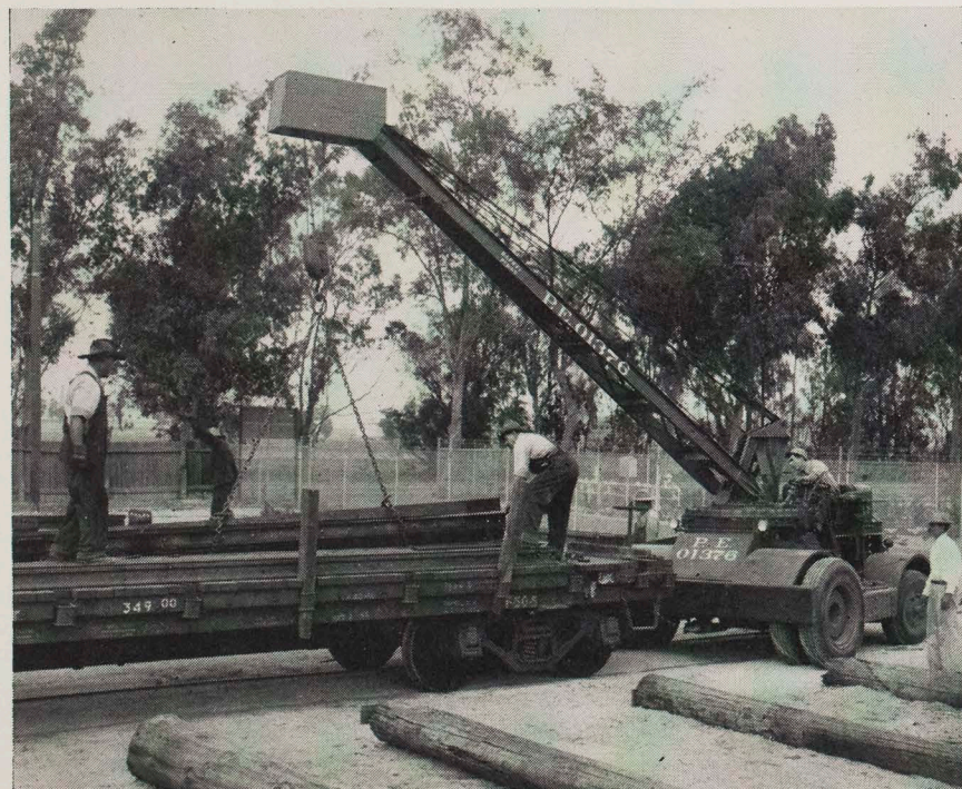
NEW CRANE—7½-ton roustabout automotive type crane purchased for the Torrance Store was placed into operation in September. Its advantages over the old rail crane are greater mobility, faster action, and greater capacity for its size, saving much valuable time.
