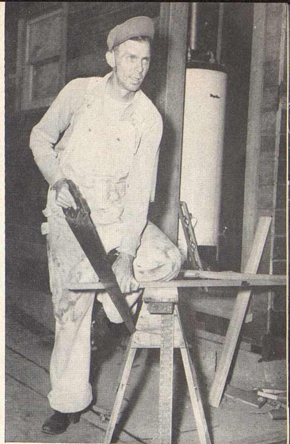
HOME-BUILDER — E. C. Hawkins , El Monte Operator, is building his home by his own labor. Corner of home is seen in background.
