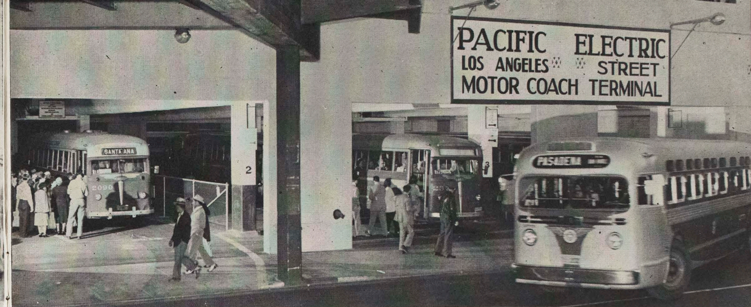
NEW LOS ANGELES STREET BUS TERMINAL, WHICH OPENED OCTOBER 9.
