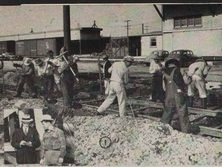
(1) Sec. 23 changing ties on team track at Long Beach Freight Station. Jose Ramirez, Subforeman, holding track level at center rear. Inset is Foreman Augustine Plasencia, right, talking to South Roadmaster L. J. Bush. (2) Sec. 30 surfacing track near La Verne, on San Bernardino Line. Foreman A. B. Holmes in left foreground. (3) Sec. 32 surfacing track at Grapeland on San Bernardino Line. Note track level across track. Subforeman Jesus Garcia at left taking over in absence of Foreman Charles Shunk. (4) Part of Extra Gang 1 cleaning off track at Harbor City after Jan. 8 rain. Foreman James E. Jeffers in white hat, third from right. (5) Main force of Extra 1 changing ties on storage track at Torrance Station. Subforeman Jesus R. Gonzales at right. (6) Extra 2 removing old yard tracks at Burbank Station. Foreman Bartolo Leyva in dark coat, right center. (7) Paving Gang 31 repairing paving at Hellman and Ramona on San Bernardino Line. Foreman James H. Carter, right. The rain was no deterrent.
