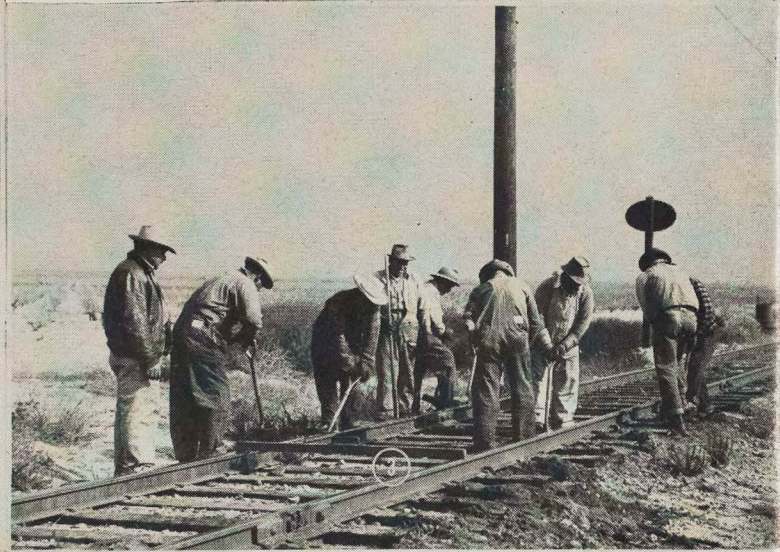
(1) Sec. 23 changing ties on team track at Long Beach Freight Station. Jose Ramirez, Subforeman, holding track level at center rear. Inset is Foreman Augustine Plasencia, right, talking to South Roadmaster L. J. Bush. (2) Sec. 30 surfacing track near La Verne, on San Bernardino Line. Foreman A. B. Holmes in left foreground. (3) Sec. 32 surfacing track at Grapeland on San Bernardino Line. Note track level across track. Subforeman Jesus Garcia at left taking over in absence of Foreman Charles Shunk. (4) Part of Extra Gang 1 cleaning off track at Harbor City after Jan. 8 rain. Foreman James E. Jeffers in white hat, third from right. (5) Main force of Extra 1 changing ties on storage track at Torrance Station. Subforeman Jesus R. Gonzales at right. (6) Extra 2 removing old yard tracks at Burbank Station. Foreman Bartolo Leyva in dark coat, right center. (7) Paving Gang 31 repairing paving at Hellman and Ramona on San Bernardino Line. Foreman James H. Carter, right. The rain was no deterrent.
