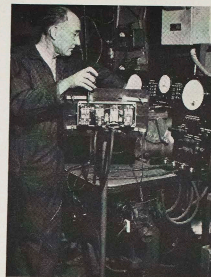
AL WHITE, Auto Machinist at Macy Garage, checks a regulator box on the test bench.
