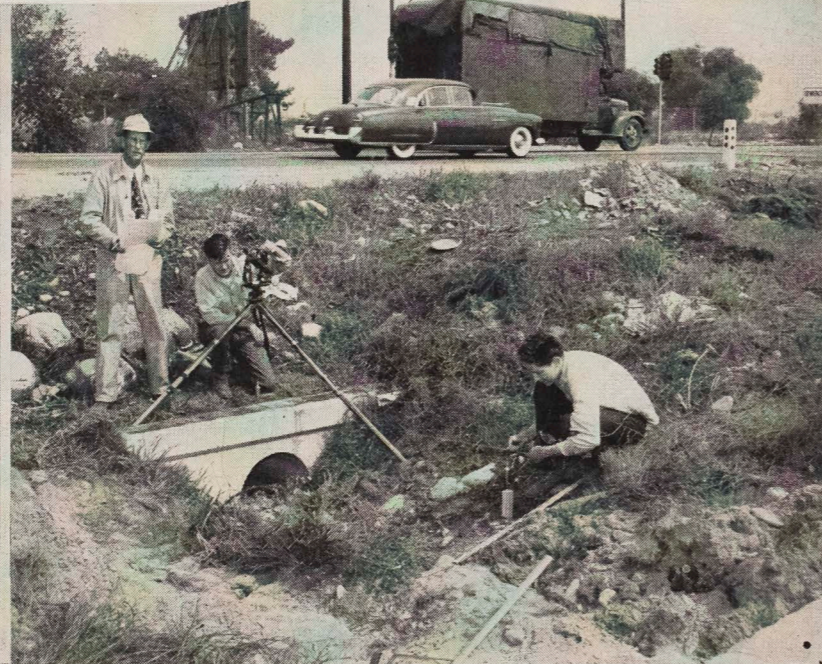
vador Arellano, on ground at left. Stacking ties at right was Anselmo Sarmiento. In car were Apolnair Contreras, Raymond Madrigal, Jose Serrano and Refugio Garcia. Considerable new track had been laid. LOWER RIGHT—Line grade for culverts under Foothill detour is being set by (left to right) C. J. Cobb, Field Engineer; Donald Knosp, Instrument Man; and Wilson Dunn, Rodman. The detour for highway traffic will be constructed so that a cut may be made in the main highway (on which car and truck are seen) in order to build underpass.
