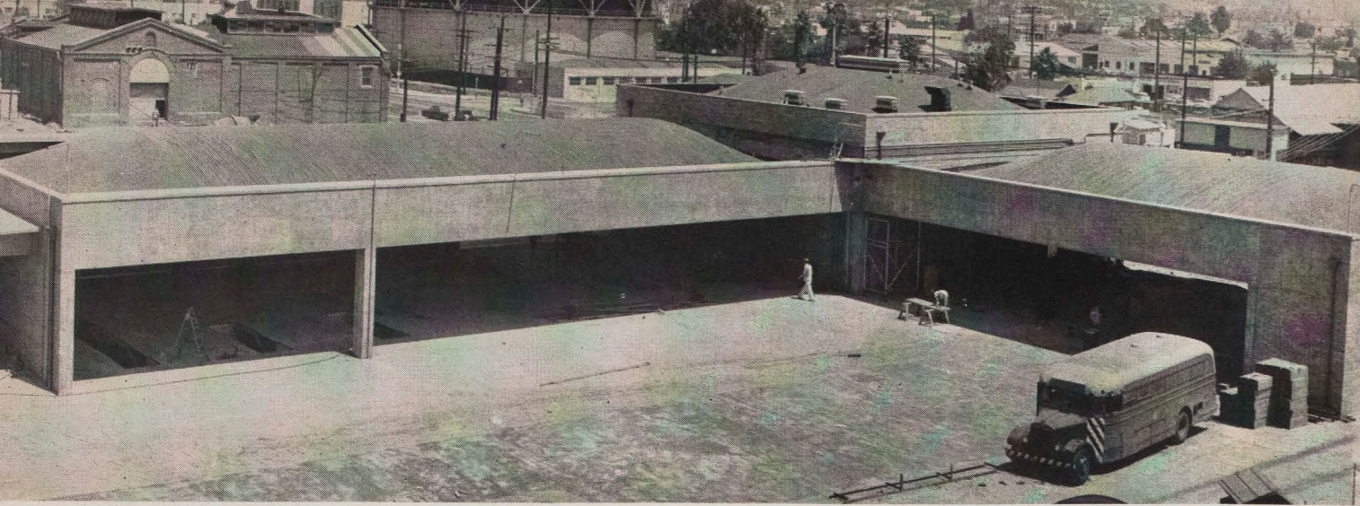
TO OPEN AUG. 25—Venice Garage as it looked Monday, July 30, from the south side. Right wing is for inspection and servicing; left, for general repairs. Note the absence of supporting columns, in the
