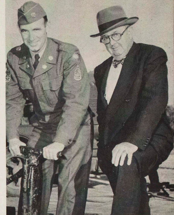
AMONG THOSE PRESENT at the "golden spike" ceremony were Field Engineer (on military leave) Wm. John Blackburn, left, and President O. A. Smith. Blackburn did the major survey work to establish alignment for present construction of connecting track between present end of former Reliance Rock Spur and Monrovia-Glendora Line at a point west of Azusa. He is now a Sergeant, 1c, in an infantry regiment.
