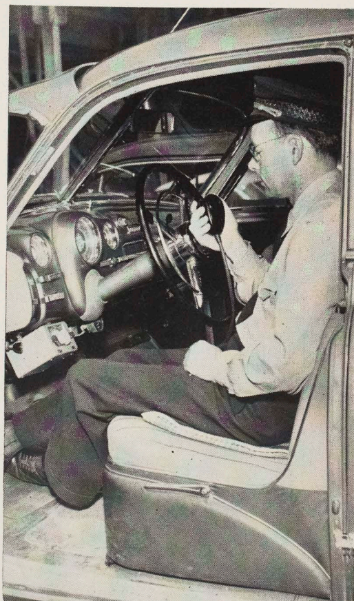
MOBILE RADIO UNIT—Harry Fowler, Motor Transit Operator, demonstrates the two-way radio set—a seven-band, 35-watt shortwave unit—which he has installed in his automobile. He has signed up for emergency civil defense communication in his home town of Whittier.
