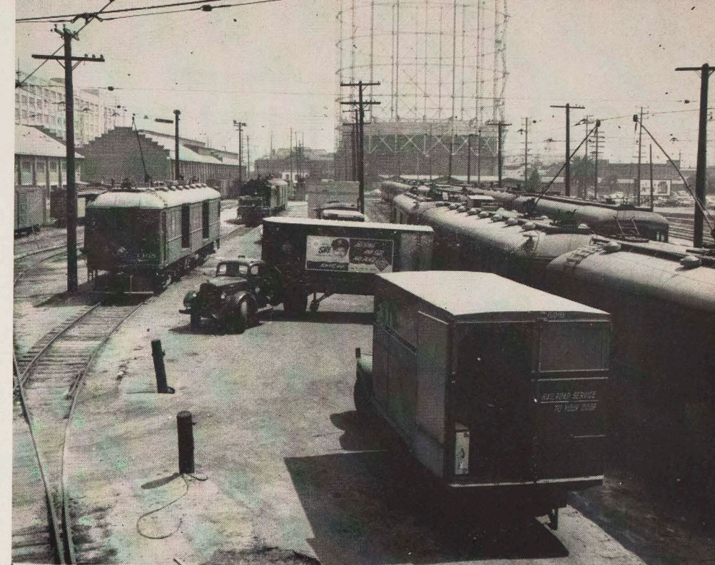
AT 8TH ST. YARD, 10 cars arrive and 10 leave daily with Railway Express Agency Shipments. This yard replaces the LAUPT as the focal point of express operations on the PE system.
