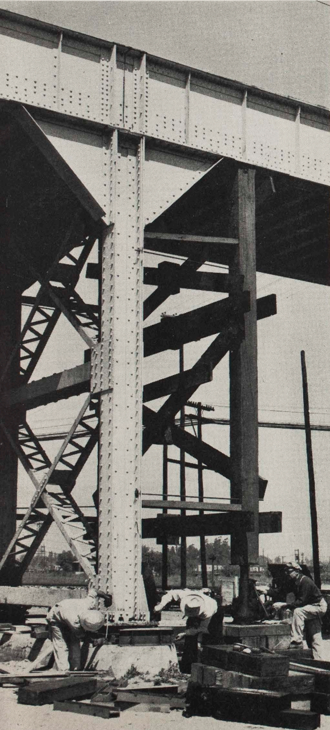
← CLOSER VIEW of one of the bridge supports, showing 100-ton jack under wooden framework near steel bents. Workmen are measuring distance bent has been raised from concrete base.
