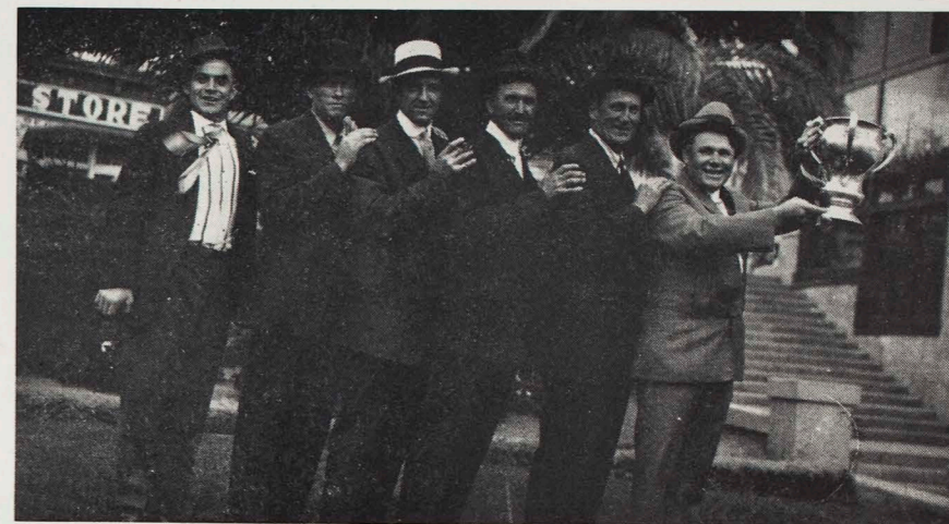
IN THE OLD DAYS—Electrical Department tug-of-war team, system champs, as snapped by a camera hound about 1916 or 1917 at the Redondo Picnic, according to retired Substation Operator E. L. Martin , a member of the team. Left to right are Owen J. Moser (now with LATL), James Truelson , Harry Widrig , Melvin Moore , Martin , and Andy Herskind (Captain). "Men used to train for the tug-of-war from May till August, when the picnic was held," says Martin . "Ten thousand people would come."
