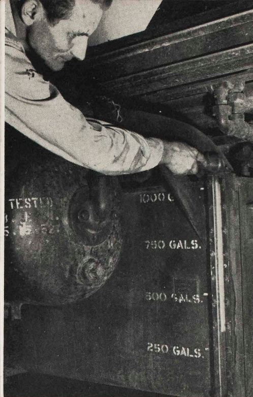
VISA-GAUGE , which indicates number of gallons of diesel fuel remaining in 1000-gallon tank, being demonstrated by Auto Machinist James E. Sisco. Lucite material carries flashlight beam along the gauge.
