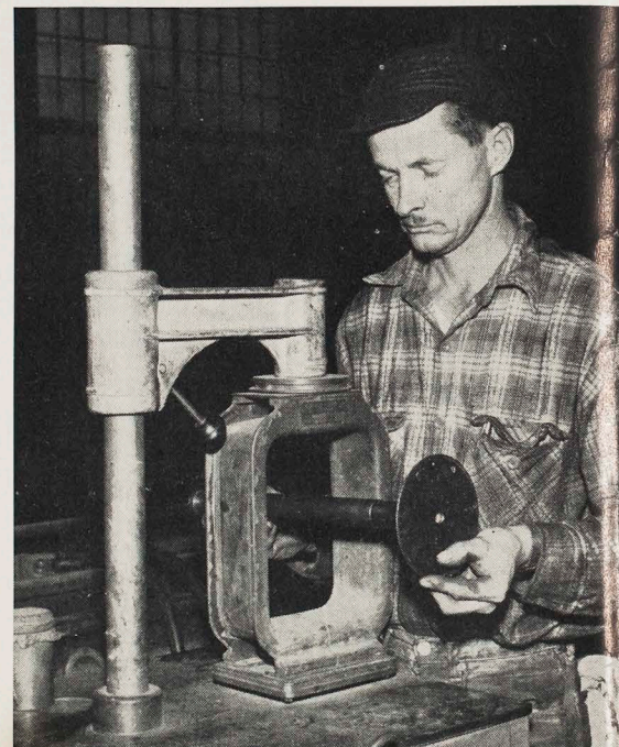
MAGNAFLUXING diesel valve for hidden defects is Auto Machinist Vernon Bliss.
