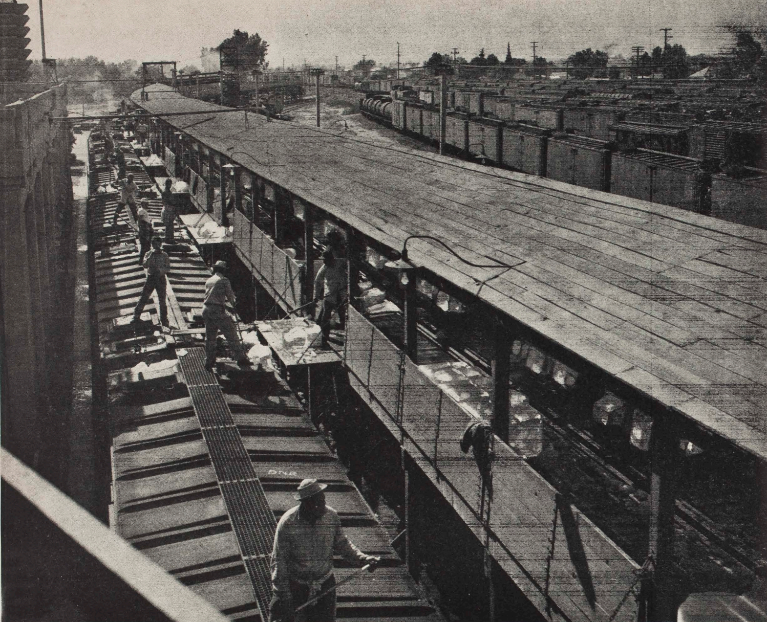
A TYPICAL ICE DOCK IN OPERATION
