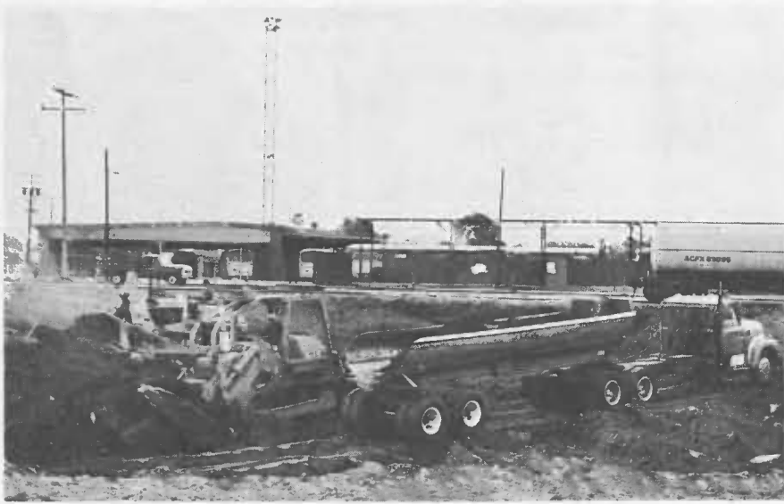
ABOVE: Overall view of the excavation work underway at the El Monte - Los Angeles Busway Station at El Monte. LEFT: Unsuitable material is removed from the building site to prepare a suitable foundation for the two-story station. The station is expected to be operational in 1973.
