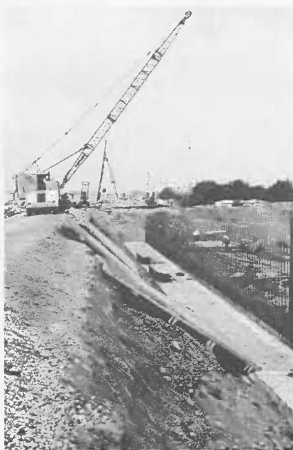
ABOVE: RTD engineers Neil Richards and Elmo Douglass talk with State engineer Jim Needham about the Busway Station beside the newly erected sign announcing the project. RIGHT: Crane lowers forms for retaining wall.
