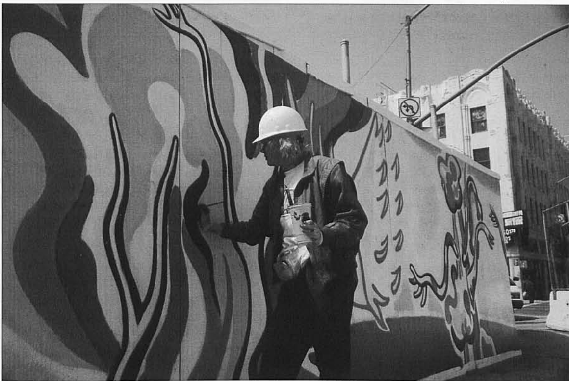
Artist Katherine Arion brings beauty to the construction fences at the Hollywood/Western Metro Red Line Station.
