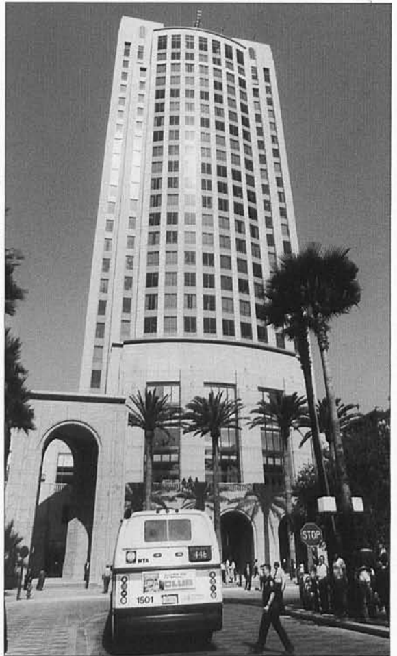
The Gateway Transit Center just received two awards that recognize the superior design of the facility.
